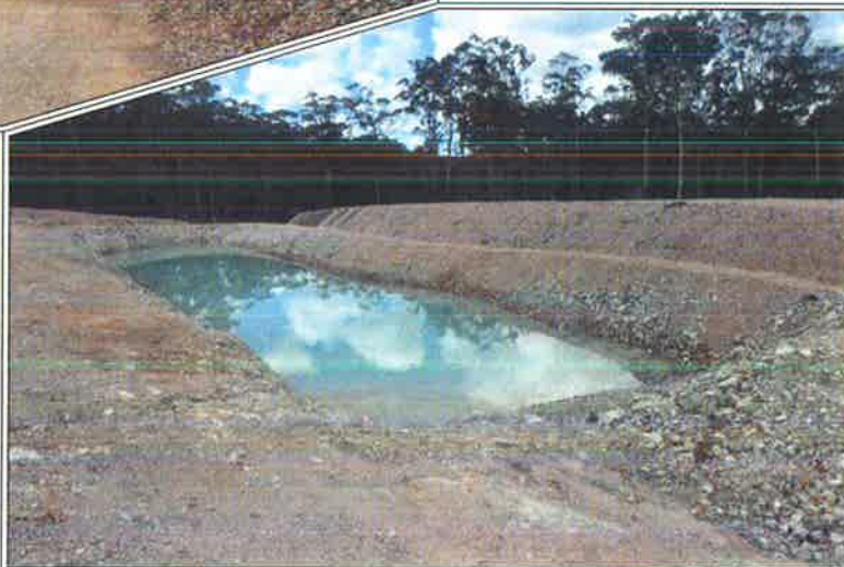
Plate 1.5: Sediment Basin D within the Extraction Area (Ref: E882F_042)
